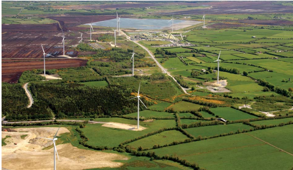
Lisheen Windfarm Project
